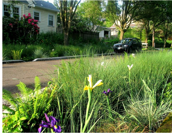
Figure 6-3: NE Siskiyou Green Street in Portland, Oregon avoided alterations to the existing storm pipe infrastructure and was therefore built cost-effectively.
