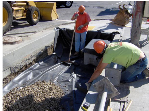
Figure 5-23: An impermeable liner is placed within a flow-through curb extension project to inhibit water migration into a nearby utility vault.
