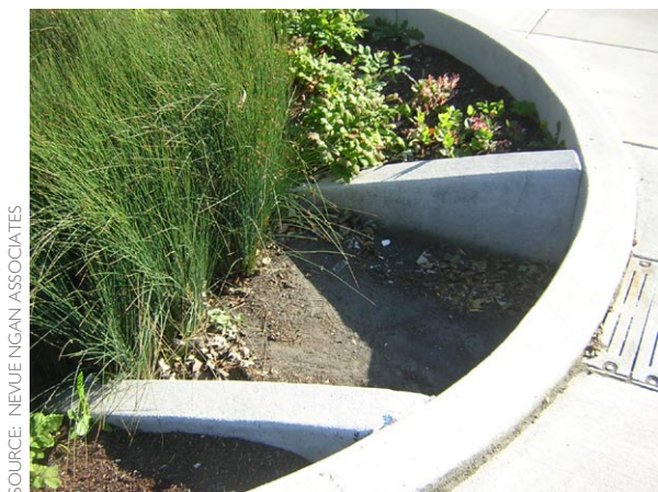
Figure 5-42: A 3x3 foot concrete pad is used as a sediment forebay for a large street rain garden. The plant material acts as a dam allowing debris to settle on the pad for regular removal.
