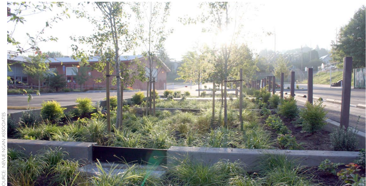
Figure 4-26: EXAMPLE: This vegetated swale utilizes check dams and adjustable weirs to control the ponding of stormwater runoff.
