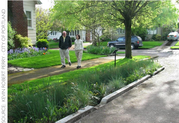
Figure 2-80: In this residential street example, runoff is completely managed within a stormwater curb extension.
