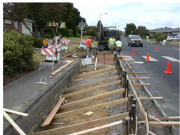
Figure 5-25: A deeper curb profile is poured along this green street project to help inhibit lateral migration of stormwater into the street’s subgrade.
