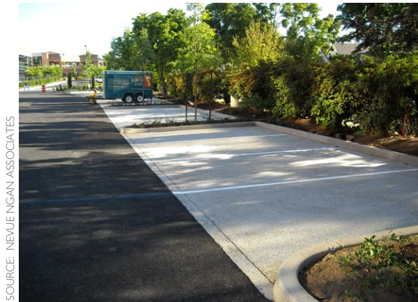
Figure 2-41: Pervious concrete allows for stormwater management and its light color helps reflect heat rather than absorb it.
