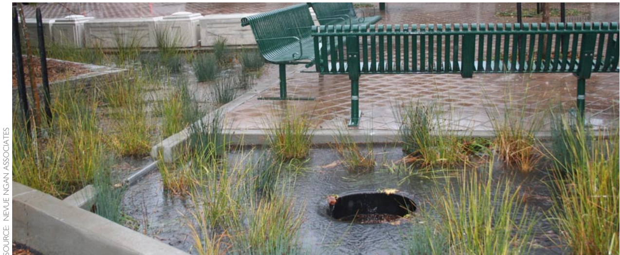
Figure 5-46: An adjustable weir retains stormwater to an 8 inch depth within this stormwater planter before overflowing into the storm drain system.
