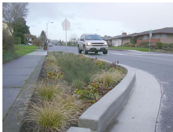
Figure 6-11: This mid-block stormwater curb extension project keeps the existing street curb in place and allows stormwater runoff to overflow back into the street without using any piped overflow structures. The combination of these strategies helped reduce construction costs.
