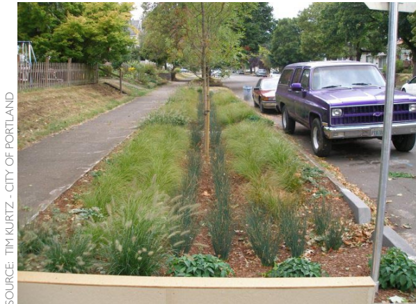
Figure 6-6: Simple green streets, such as this residential example in Portland, Oregon, convert under-utilized landscape area next to streets into stormwater facilities. Since the improvements consist largely of regrading and planting, the projects can be very cost effective to build.
