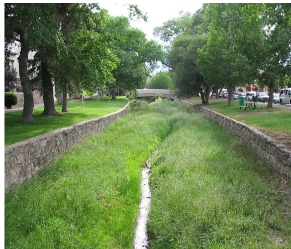
Figure 2-25: Vegetated channels like this can be designed even in urban conditions for the purpose of conveying stormwater runoff.
