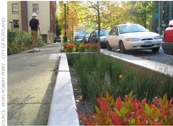
Figure 2-58: An urban street infiltration planter.
