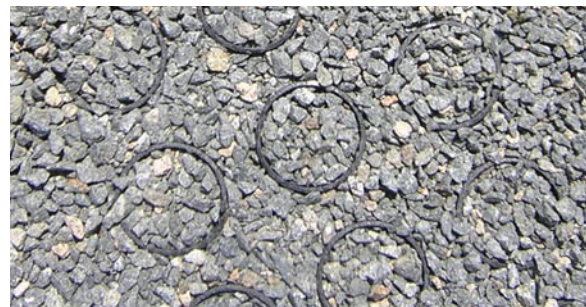
Figure 2-45: A close up view of gravel paving within a reinforced plastic grid system.
