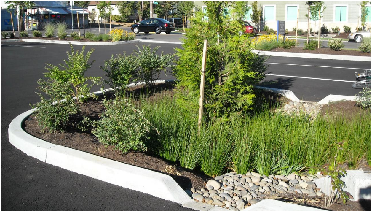
Figure 4-56: EXAMPLE: This parking lot treats a portion of its stormwater runoff within multiple stormwater planters.
