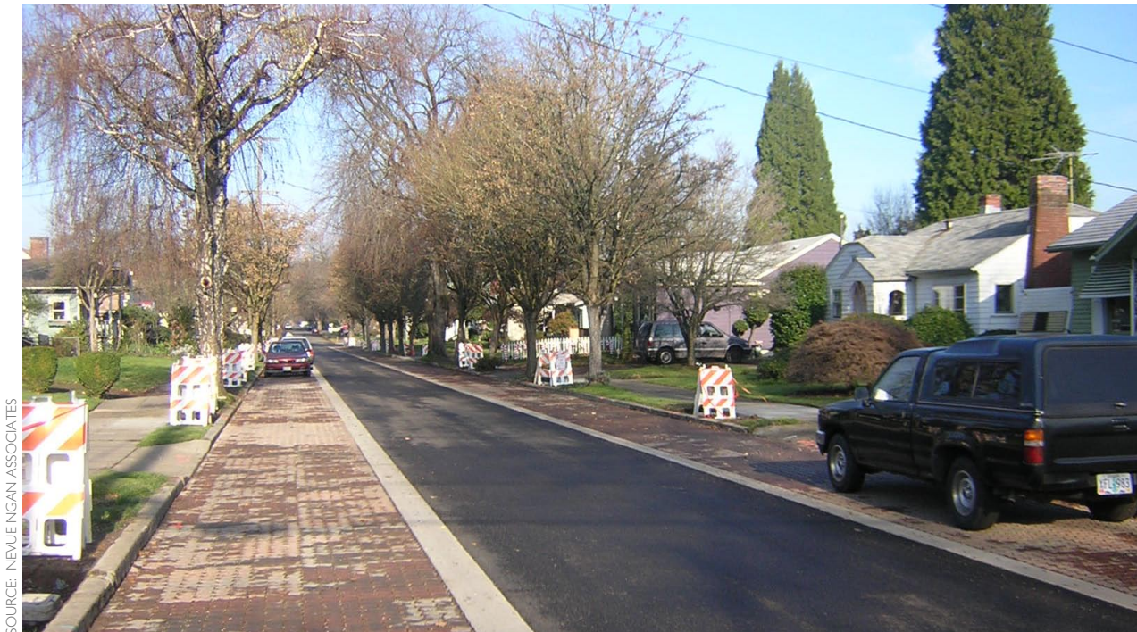
Figure 4-20: EXAMPLE: Concrete pavers used in a residential street's parking zone. Notice the visual "narrowing" of the street.
