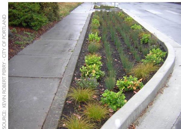
Figure 2-86: A stormwater curb extension along a neighborhood collector street. For this project, the existing street curb was retained.
