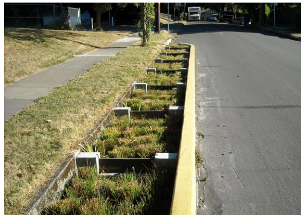
Figure 6-5: This stormwater curb extension project constructed in Portland, Oregon reduced project costs by leaving the existing street curb in place.
