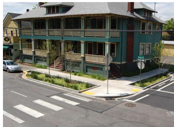
Figure 2-89: An urban intersection retrofitted with stormwater curb extensions.
