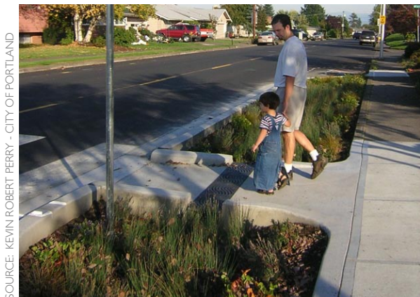
Figure 2-87: Curb extensions can provide for stormwater management and safer crossings for pedestrians.
