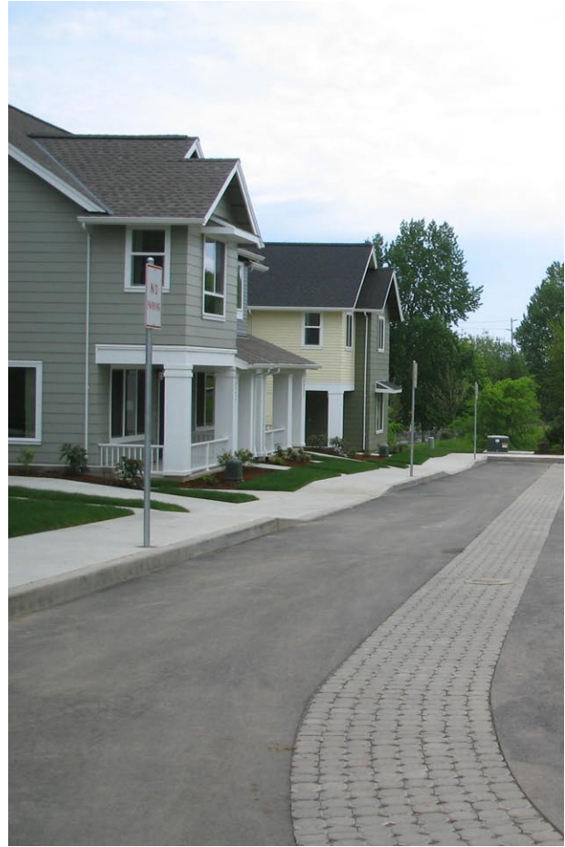
Figure 4-30: Sand-set concrete pavers installed in the center strip of a multi-family housing driveway approach.
