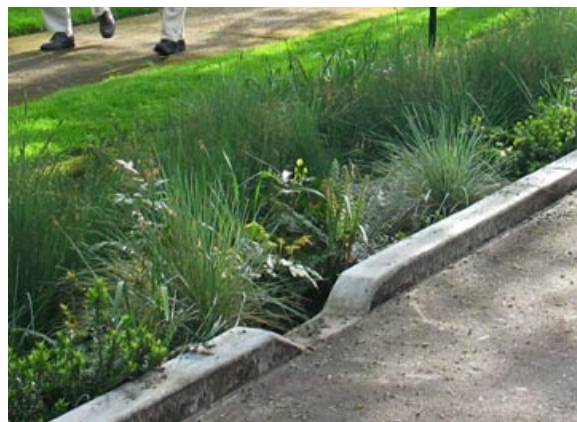
Figure 6-10: In contrast to the example above, a simple cost-effective curb cut allows water to move freely into a stormwater facility without detracting from the aesthetics of the project.
