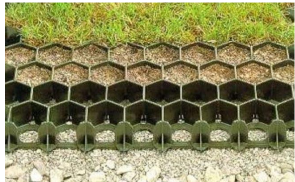
Figure 2-39: Reinforced grass paving allows water to pass through the root zone of the grass and into the underlying soil while still maintaining a hard surface for vehicular travel.
