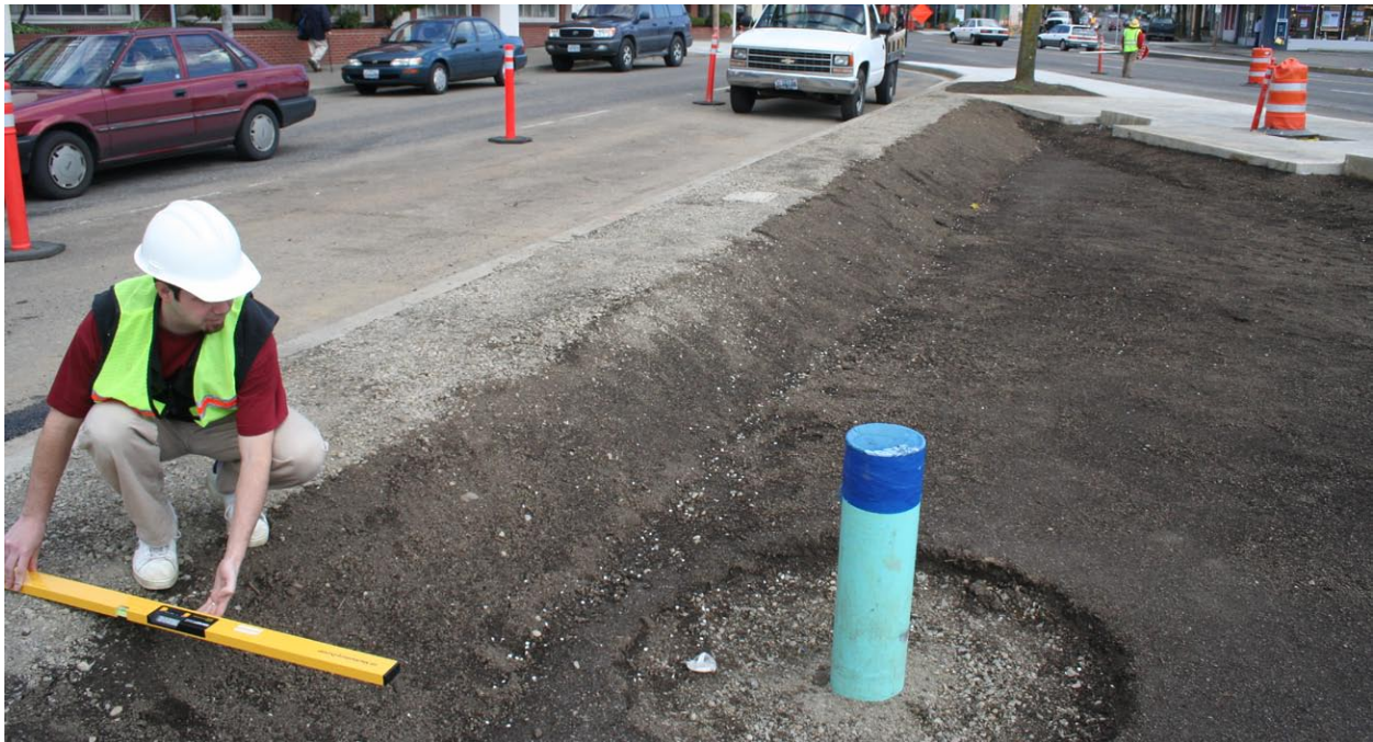
Figure 5-56: The design team should be on-site regularly during the grading process to determine whether or not the grading is consistent with the plans, and if necessary, work with the contractor to make field adjustments.
