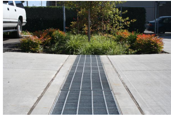
Figure 5-37: This trench drain example connects two stormwater facilities within an industrial parking lot site.
