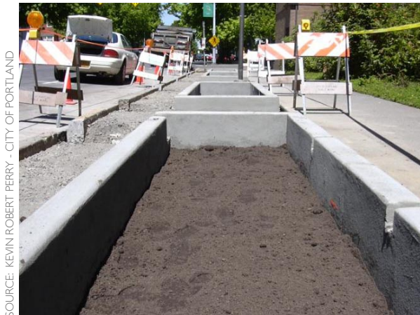
Figure 5-52: New imported topsoil is placed within a planter. Soil is graded 2 inches lower than finish grade to allow for a mulch layer.
