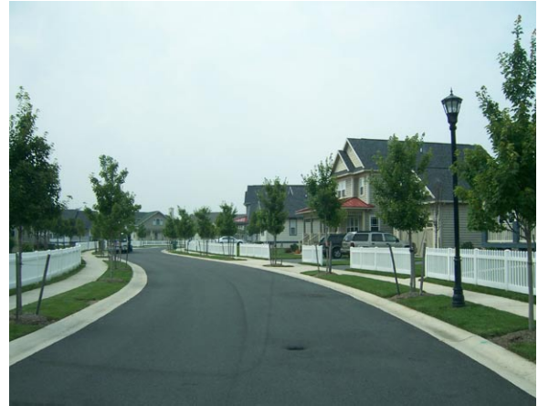
Figure 4-14: EXISTING: A residential street within a new development project.
