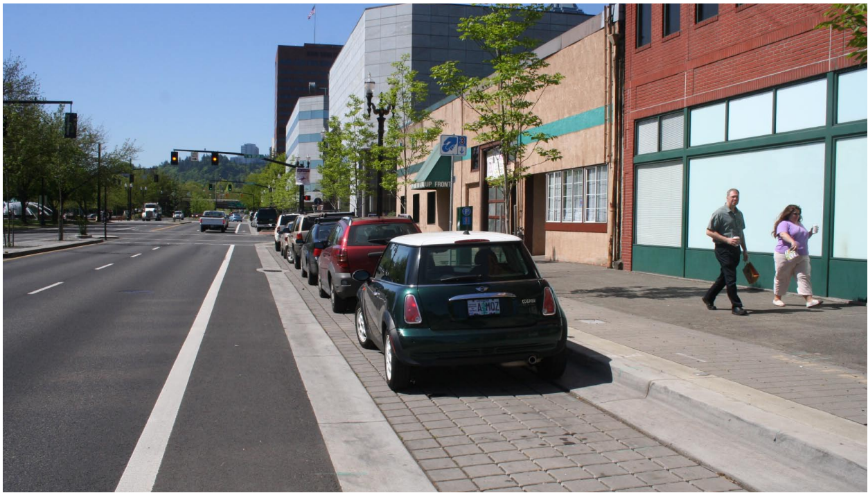
Figure 4-41: EXAMPLE: This urban street uses pervious paving in its parking zone and could have been further refined with stormwater curb extensions.
