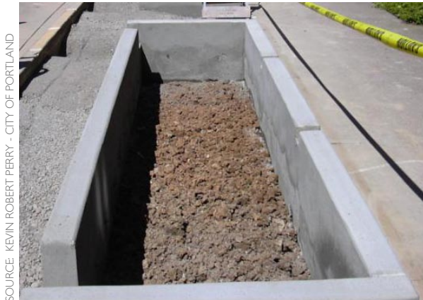
Figure 5-51: Native soil is rototilled to break up construction compaction.
