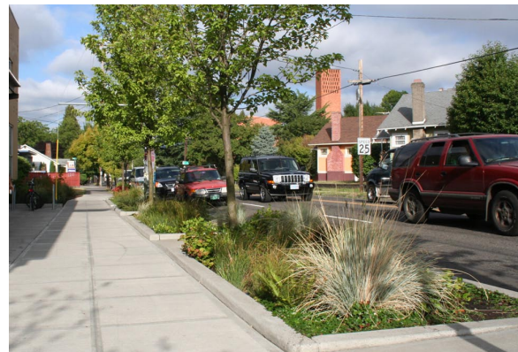
Figure 6-12: This green street project built in 2004 in Portland, Oregon was a first-of-its-kind on a commercial street. Demonstration projects like this one have helped spur other green street projects, as well as provided the impetus for changing municipal design standards and codes.
