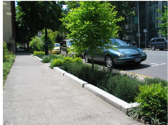
Figure 6-17: Portland's SW 12th Avenue Green Street project utilizes a strategic approach in placing smaller stormwater facilities intermittently along the streetscape.
