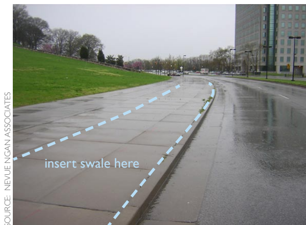
Figure 2-51: A potential urban street swale opportunity in an overly wide sidewalk zone. Dashed lines show where a vegetated swale could be added.
