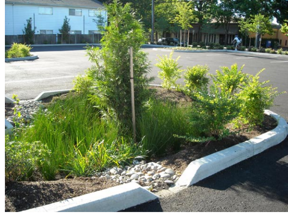
Figure 2-66: A stormwater planter within a parking lot's landscape island.
