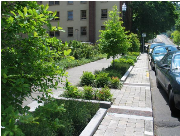
Figure 2-64: Stormwater planters located on a street with on-street parking.
