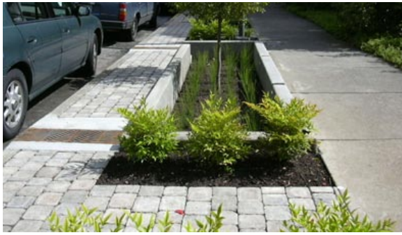
Figure 5-10: This street utilizes stormwater planters adjacent to on-street parking. It provides a continuous 3-foot pedestrian egress zone and walkways that allow people to access the sidewalk and parking zone.
