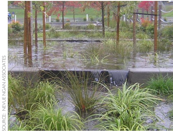
Figure 1-9: Stormwater facilities slow the flow of stormwater runoff through the interaction of the water with plants and soil.
