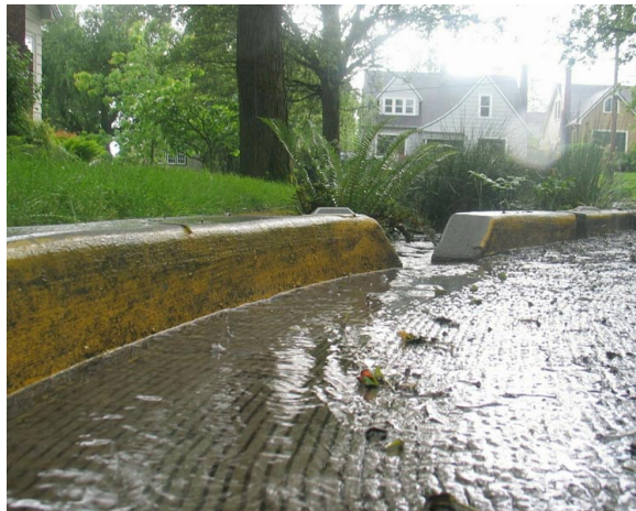
Figure 5-27: A typical curb cut used to allow water to enter a stormwater curb extension.
