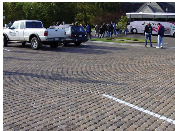
Figure 1-22: Light-colored pervious paving within a parking lot helps reflect heat rather than absorb it.
