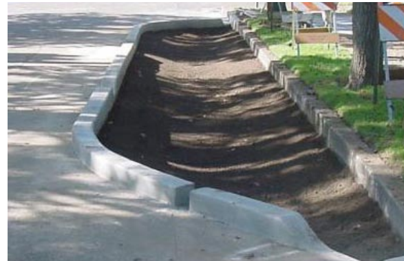
Figure 5-54: A shallow graded stormwater curb extension retains a maximum of 7 inches of water.
