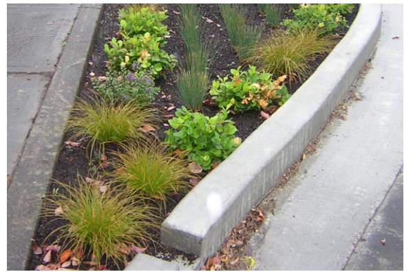
Figure 5-45: Overflow from a mid-block stormwater curb extension exits from a curb notch and flows back onto the street.
