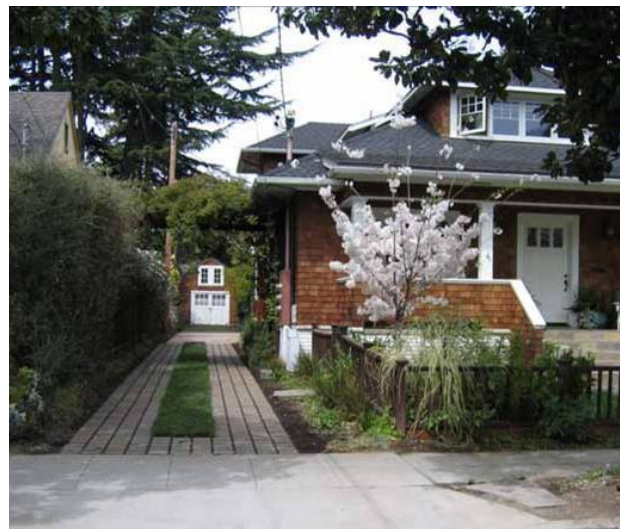
Figure 4-31: A combination of grass and pervious concrete pavers replaced a conventional driveway in Palo Alto, CA.
