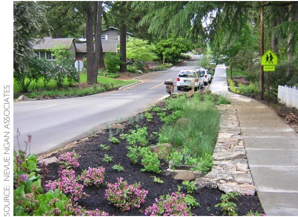
Figure 2-52: Residential street with a vegetated swale.
