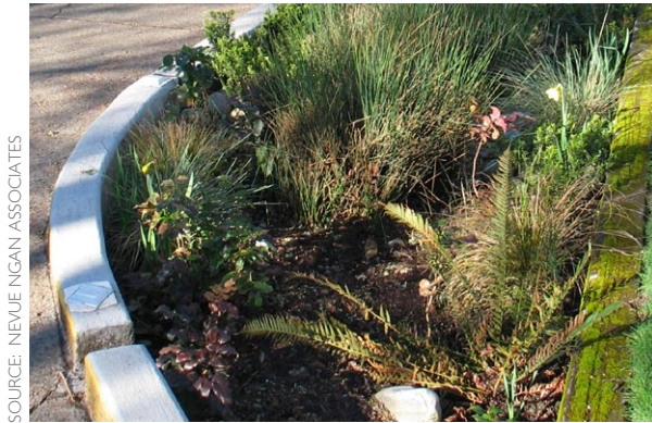
Figure 5-40: A sediment forebay within a stormwater curb extension.
