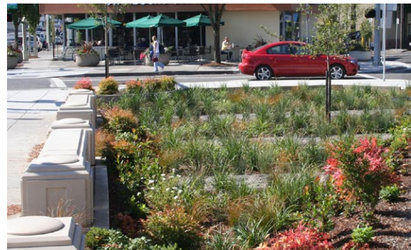
Figure 2-5: Selecting stormwater facilities, such as this rain garden, is the final step in the 3-step design process.
