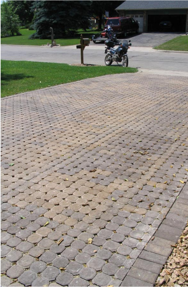
Figure 4-28: Sand-set concrete pavers installed within a driveway.
