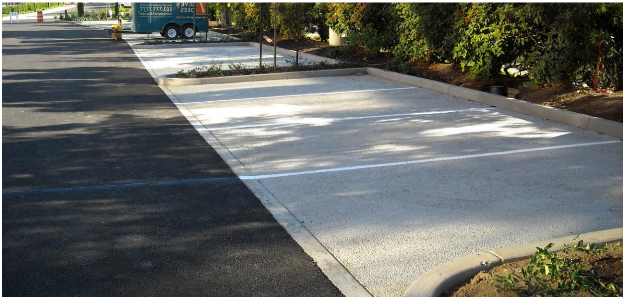
Figure 4-59: EXAMPLE: This new parking lot utilizes pervious concrete within the parking lot's parking stalls.
