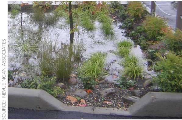
Figure 5-43: This curb cut serves as the only overflow within an infiltration rain garden.
