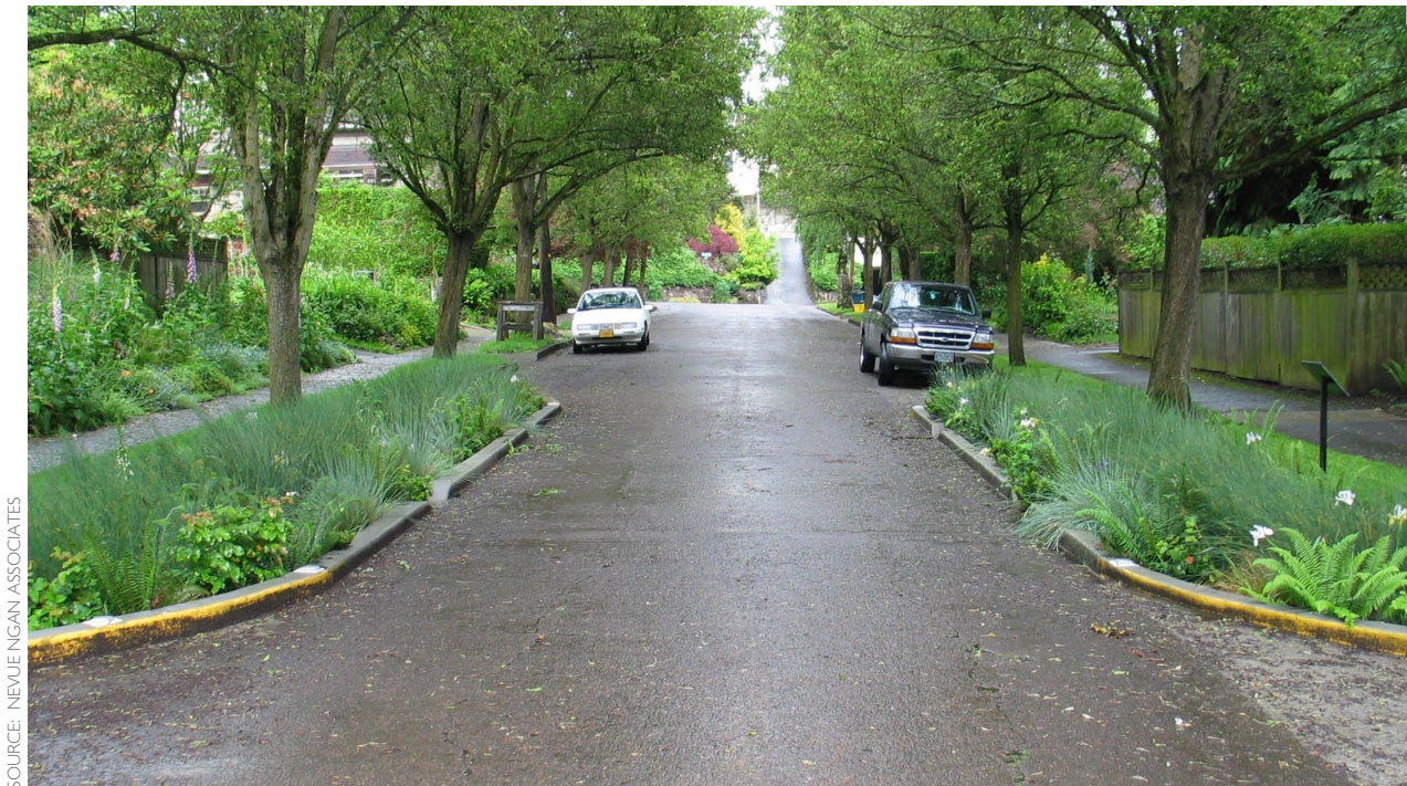
Figure 4-7: EXAMPLE: A pair of stormwater curb extensions used in a residential street's parking zone. Notice that there is still plenty of on-street parking available.
