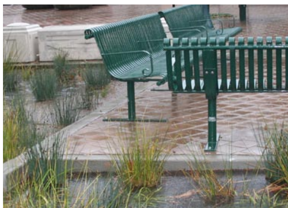
Figure 5-28: Sheet flow of stormwater runoff enters a vegetated swale from a public plaza space.
