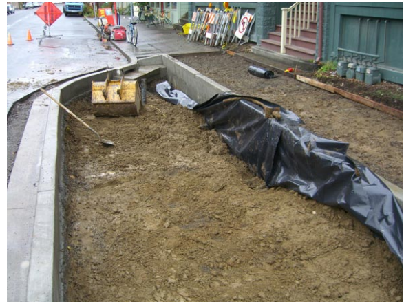
Figure 5-24: An impermeable liner is placed along the sidewalk side of an infiltration stormwater curb extension in order to protect the foundation of an adjacent building.
