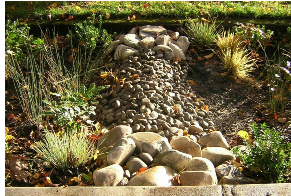
Figure 5-20: Simple checkdams made of stacked rocks or gravel can be used on gently sloped stormwater facilities.
