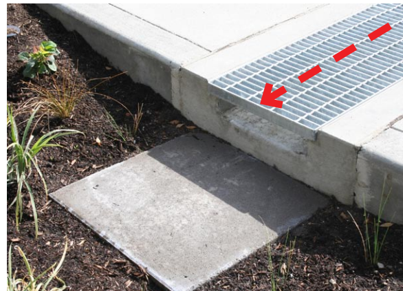
Figure 5-38: A concrete unit paver is placed at the exit point of this trench drain. The pad helps prevent erosion by dissipating water velocity as water drops from the trench drain to the finish grade of the stormwater facility.
