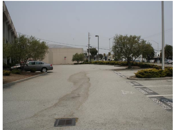
Figure 4-57: EXISTING: A typical internally drained parking lot in San Mateo County.
