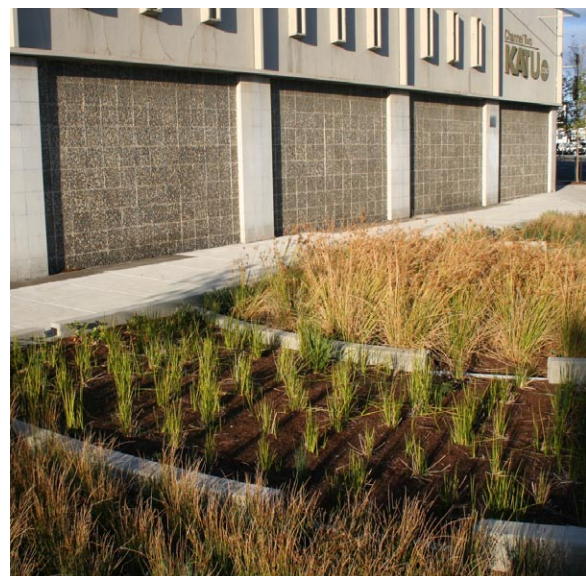
Figure 5-58: Standard bark mulch is applied to a green street project.
