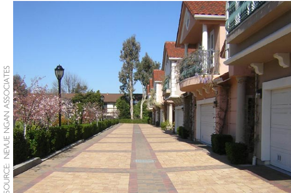
Figure 4-27: This residential development in San Mateo County utilizes sand-set concrete pavers.
