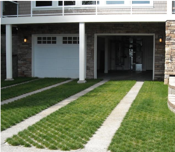
Figure 4-29: Reinforced grass paving with wheel base concrete bands.
