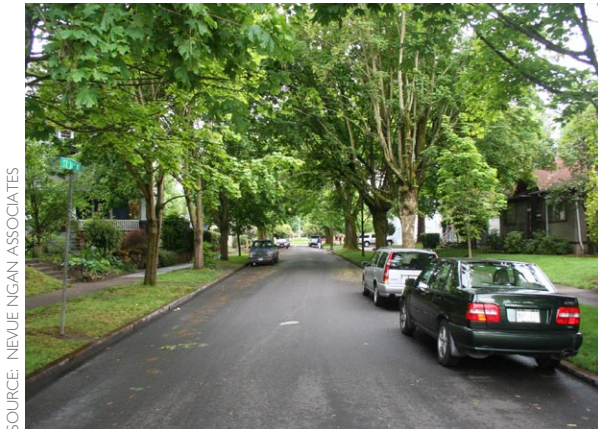
Figure 2-6: This narrow residential street allows for adequate traffic flow and generates less stormwater runoff than conventionally wider streets.
