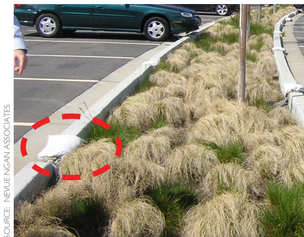
Figure 5-53: Sand bags are placed in front of curb cut inlets in order to help protect soil and plant material immediately after planting.
