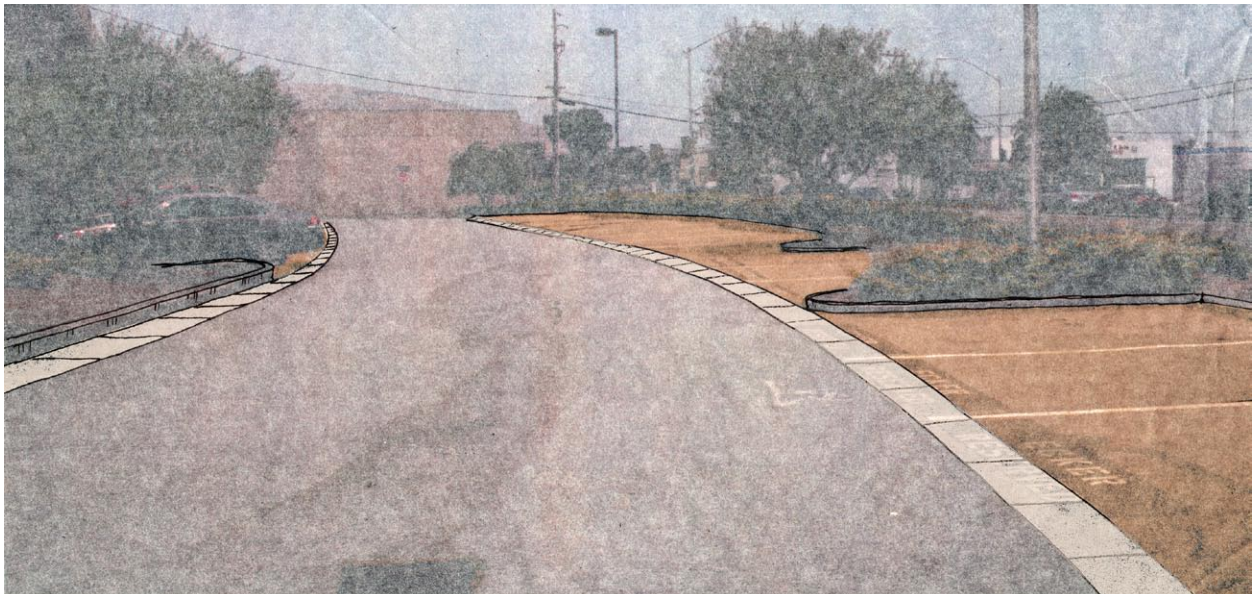
Figure 4-58: RETROFIT OPPORTUNITY: The same parking lot retrofitted with pervious paving in the parking stalls.
