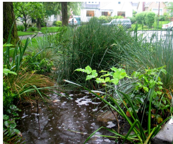
Figure I-20: Landscape-based stormwater facilities, such as this stormwater curb extension, can capture urban debris before it gets into creeks and other waterways.
