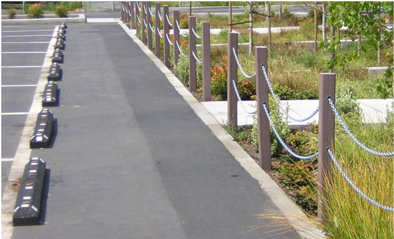
Figure 4-62: EXAMPLE: This parking lot was retrofitted with a stormwater swale with pedestrian crossings.
