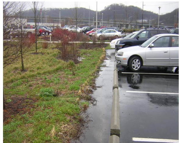
Figure 2-79: A simple grassy rain garden with trees collects runoff from adjacent parking lot stalls.
