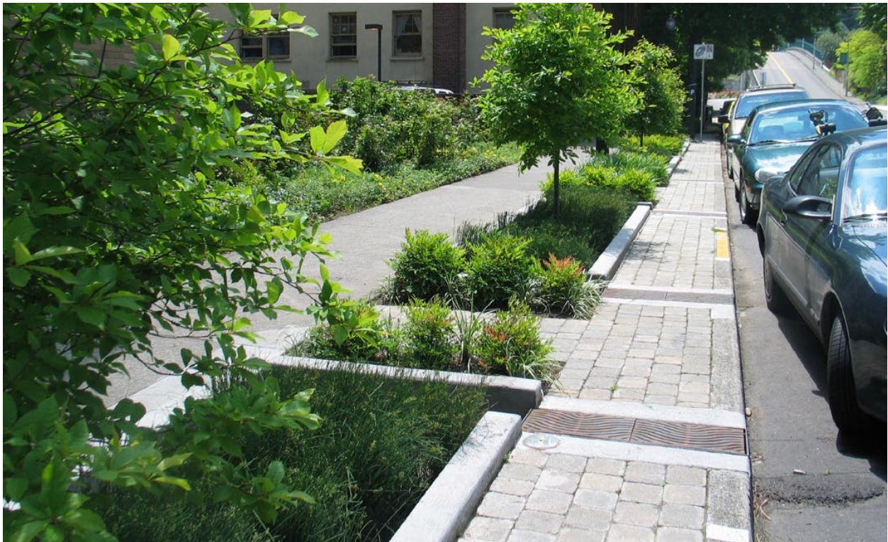
Figure 4-34: EXAMPLE: Stormwater planters used along a downtown street. Notice that there needs to be adequate space allocated for people to get in and out of their vehicles and access the sidewalk zone.
