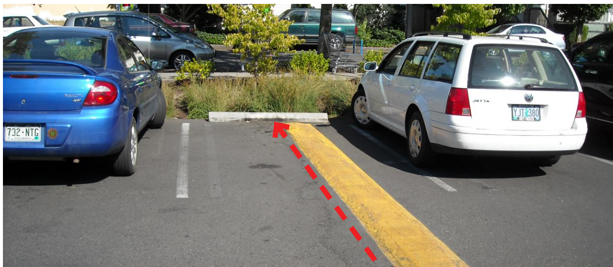
Figure 5-39: This asphalt speed bump redirects stormwater into a vegetated swale. Without the speed bump in place, stormwater runoff would enter the vegetated swale much lower within the system, bypassing some of the area available for treatment.
