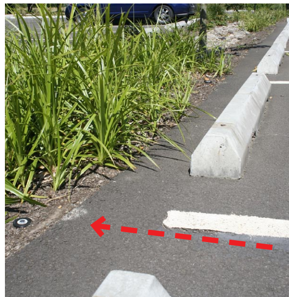
Figure 5-35: The 3 foot space in between these wheelstops allows stormwater runoff to enter a vegetated swale within a parking lot. This design could be improved by including more of a drop in grade between the asphalt and the landscape area.
