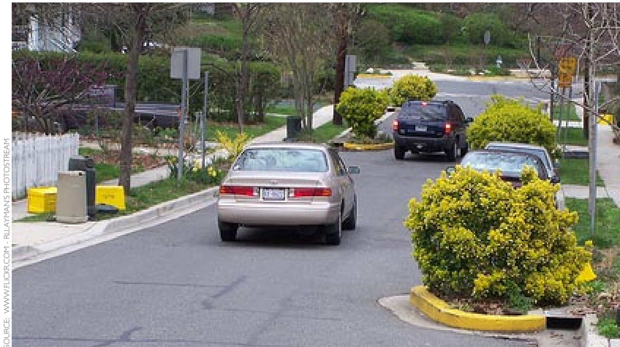
Figure 4-23: EXAMPLE: Conventional curb extensions are placed in a staggered orientation on this residential street. Although these curb extensions do not allow stormwater runoff to soak into the ground, they could be modified to do so.
