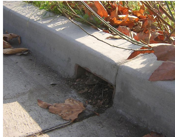
Figure 5-29: Bad example - a notched curb cut is way too small and constantly overloaded with sediment.
