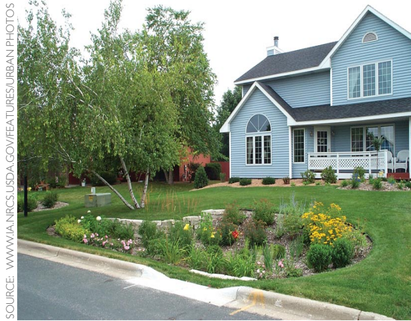
Figure 2-74: A simple residential street rain garden.
