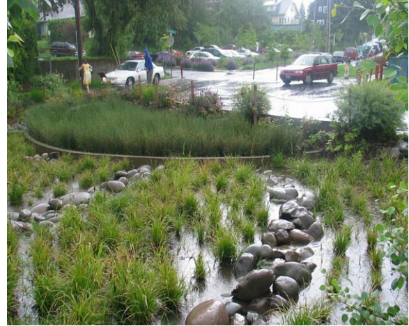
Figure 2-77: This rain garden next to an elementary school collects runoff from adjacent neighborhood streets and the school's parking lot.
