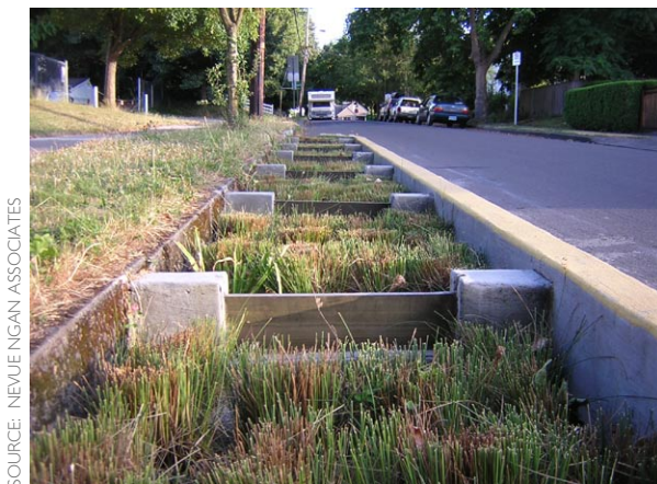
Figure 5-18: Closely spaced check dams help terrace the interior landscape of this stormwater curb extension project. The slope of this street is approximately 6%.
