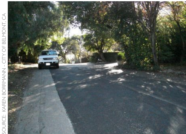
Figure 6-25: The existing conditions on Holly Road include a steep street slope, a narrow right-of-way, irregular driveway locations, and several mature street trees at the roadway's periphery.
