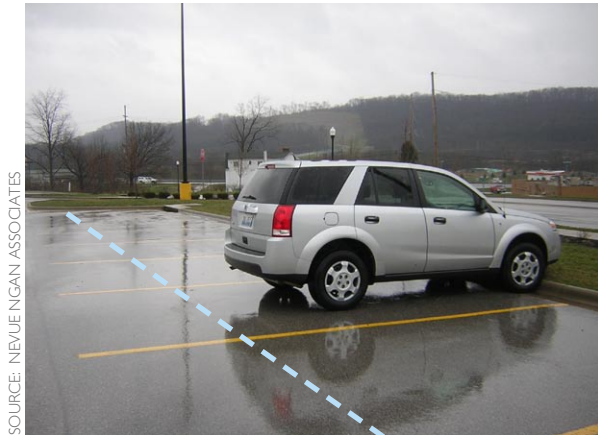
Figure 2-49: These oversized parking spaces could be made just a few feet shorter in order to create space for swales between rows of parked cars.
